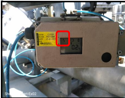
AV111 air instrument leakage, both air tube having air against which giving PCV214 default status required repairing
